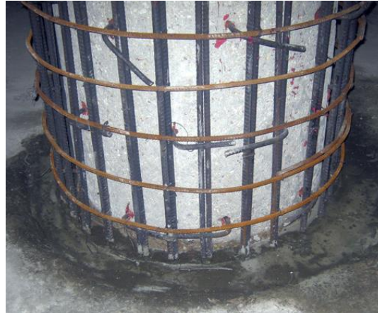
Concrete jacking
